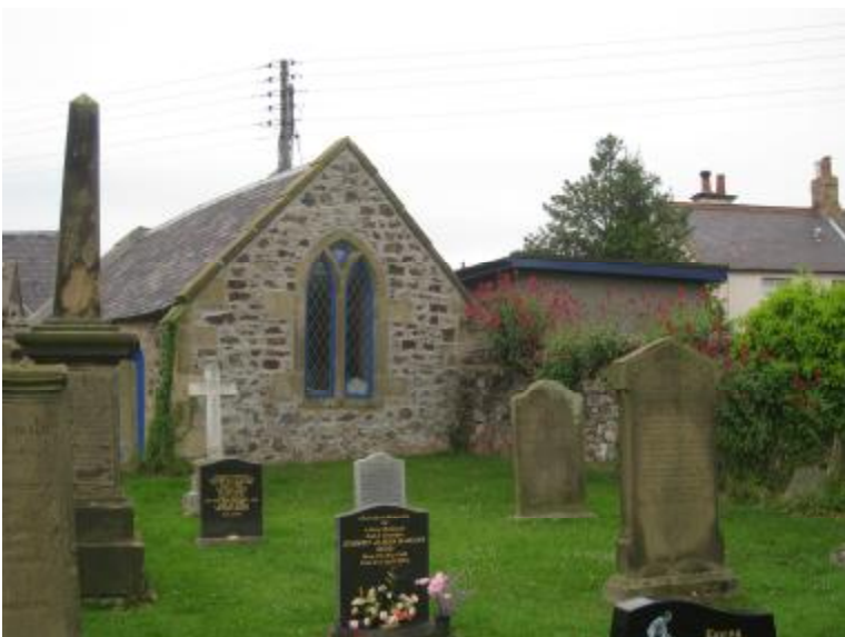
The rear of the group with the flat roofed toilet building on the right
