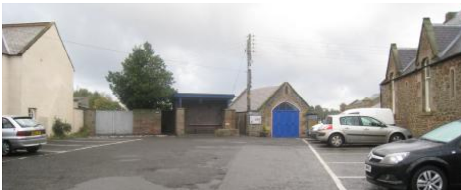
The existing building group from the Square car park
